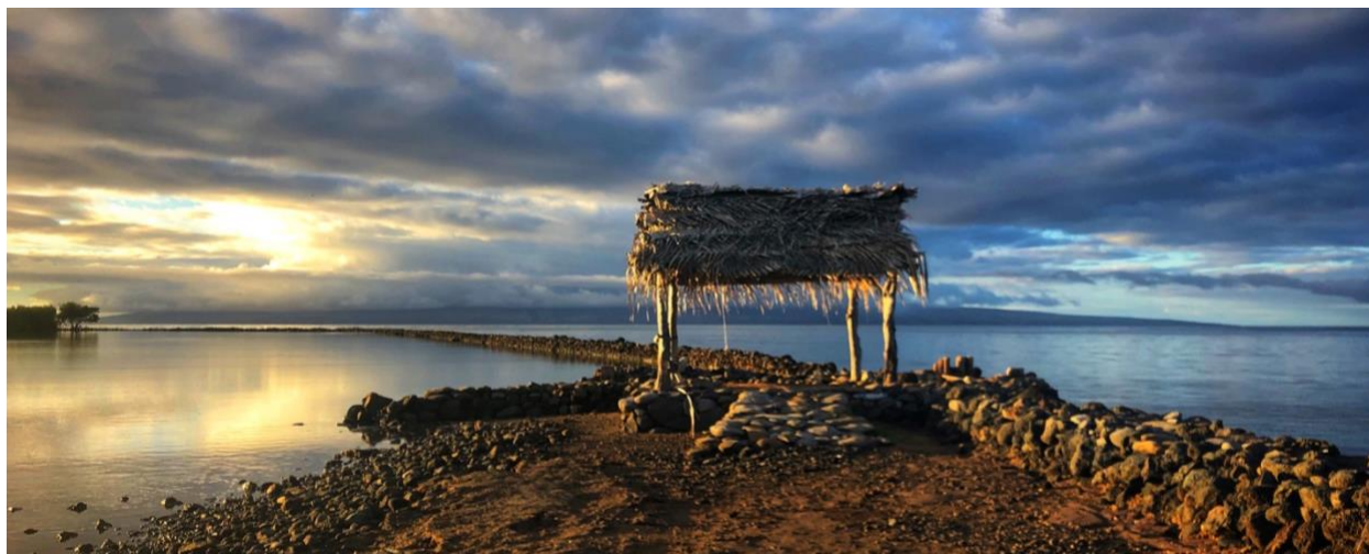
Ali'i loko i'a is a centuries-old, traditional Hawaiian fishpond on the island of Moloka'i. The watch house (kia'i) sits on the fishpond wall (kuapā) near one of the gates (makahā or "eye that breathes") through which small fish can easily enter to find refuge. Photo: Noelani Lee
